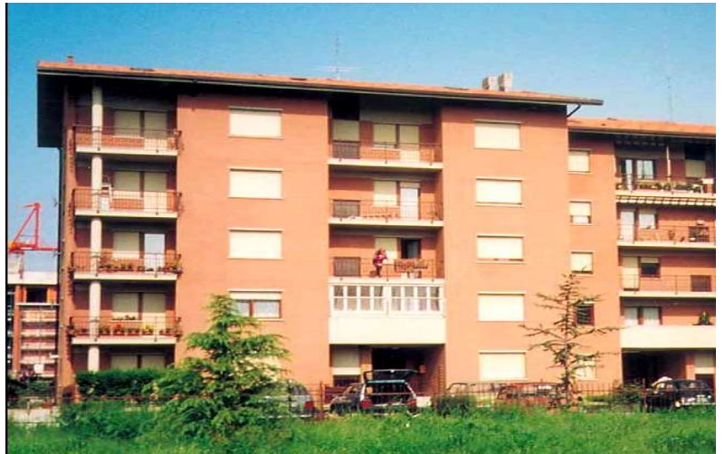
“Cedit” Condominium Collegno (TO), Italy 1990
