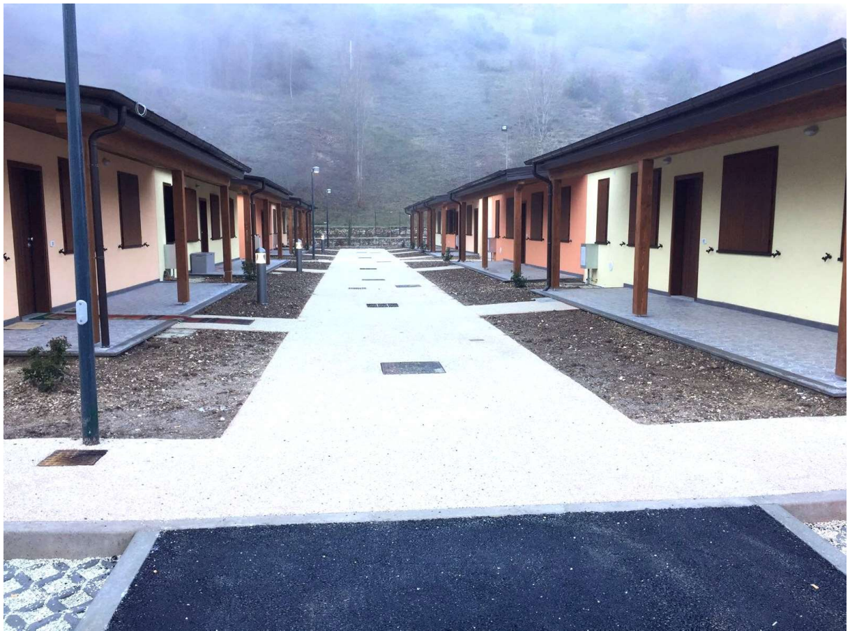
Construction of emergency houses SAE 350 in the earthquake zone of Marche, Italy Visso, 2017 / 2018
