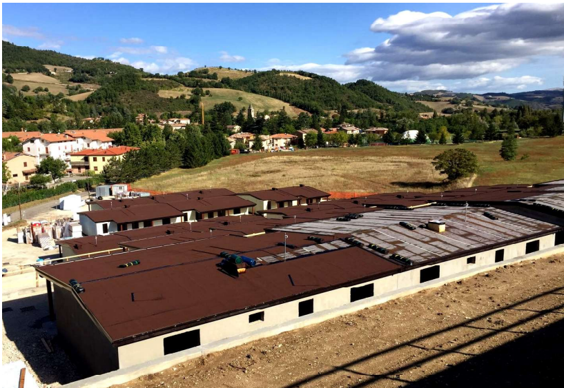
Construction of emergency houses SAE 350 in the earthquake zone of Visso, Pieve Torina, Caldarola, San Severino Marche 2017 / 2018
