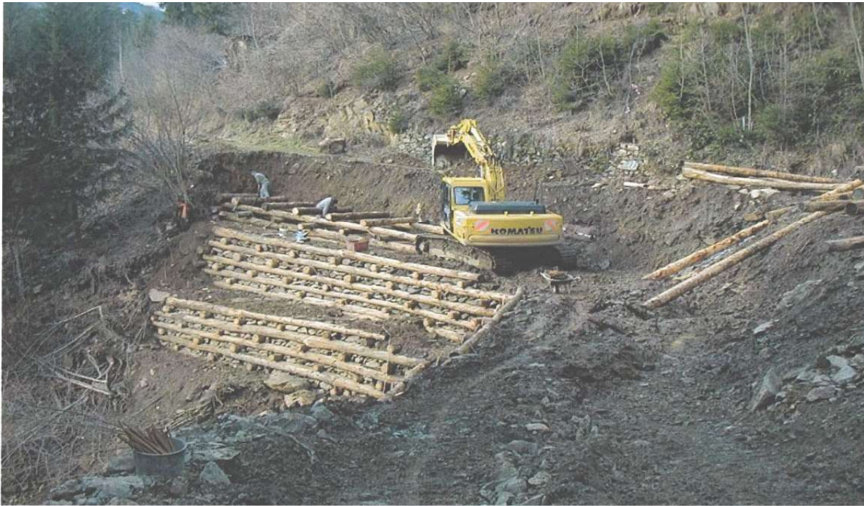
Highways works San Romolo – Bajardo, Italy 2003
