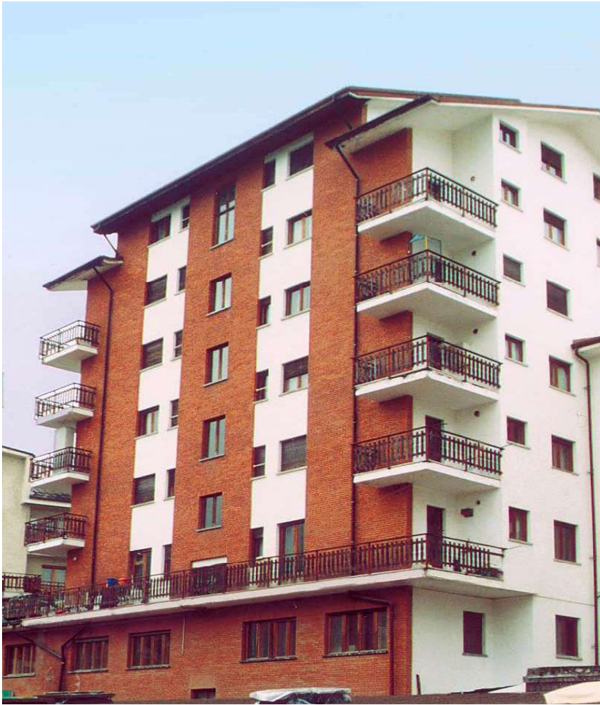
Building in Assietta Square Saule D'Oulx (TO), Italy 1965
